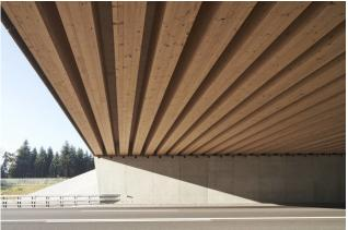
In Neuenkirch, the Federal Roads Office FEDRO is already building the second wildlife bridge with a wooden overpass after the Rynetel wildlife bridge. The wildlife overpass in the canton of Lucerne has a width of 50 meters and a length of around 36 meters.
