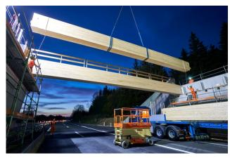
...and are placed in one piece on the concrete foundations.
