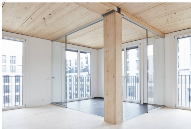
Loggia with supports and ceilings in timber construction
