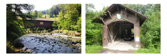
The Sihlmatt wooden bridge has connected the cantons of Zug and Zurich since its construction in 1849-1850. Timbatec Holzbauingenieure AG has determined by means of a condition survey that the bridge urgently needs to be rehabilitated and subsequently supervised the repair project.
