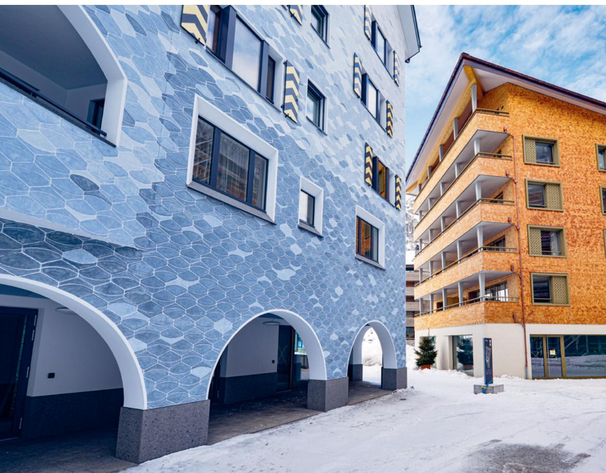
The shingle façade made of larch wood, constructed for a six-story apartment building in Andermatt was only possible due to fire tests and plans carried out by Timbatec.
