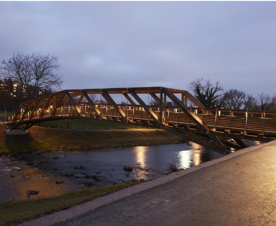
**A flagship project: the 45-metre-long Tüfisteg bridge made of Swiss beech wood**
